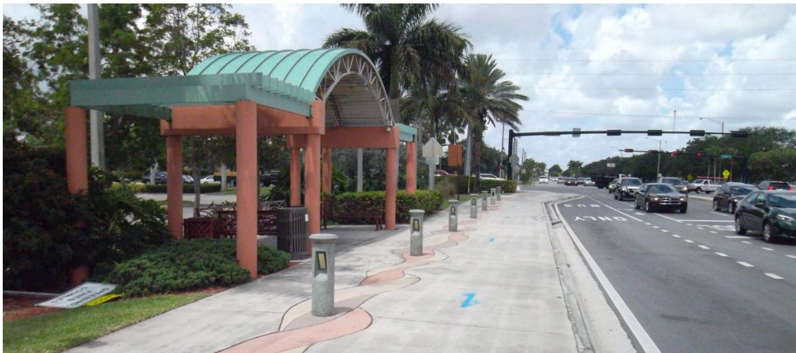
Figure 3-3: Coconut Creek Photo – Bus Shelter
