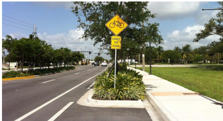
Figure 2-4: Pompano Beach – Share the Road Bicycle Facility
