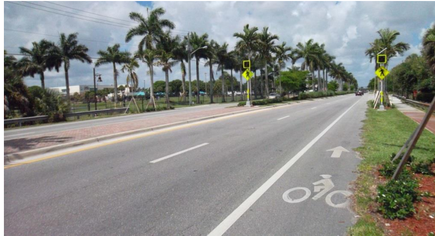
Figure 2-3: Coconut Creek – Marked Bicycle Lane
