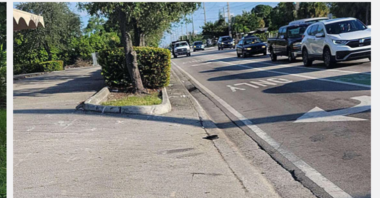
Missing sidewalk near Broward Blvd intersection
