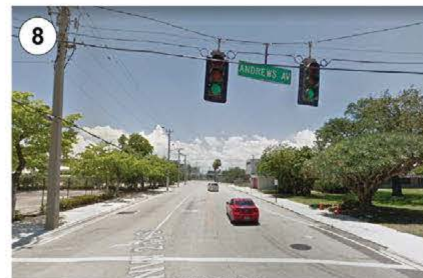
8 NW 2ND ST LOOKING WEST
