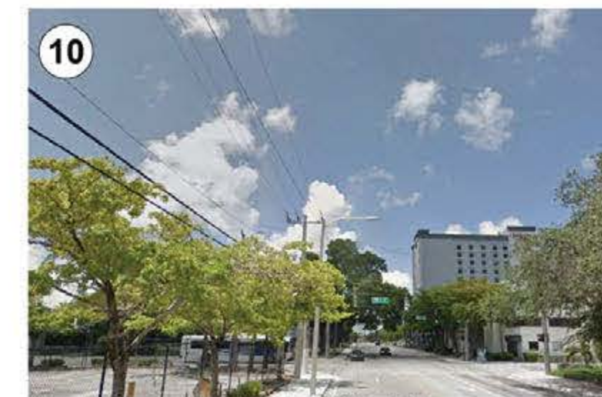
10 N ANDREWS AVE LOOKING NORTH
