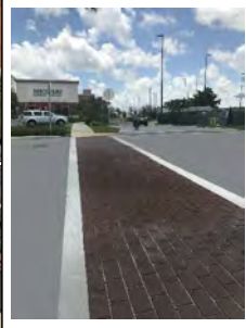
STAMPED ASPHALT CROSSWALKS
