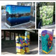
UTILITY BOX GRAPHIC WRAP
