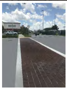
STAMPED ASPHALT CROSSWALKS
