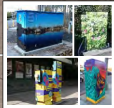
UTILITY BOX GRAPHIC WRAP
