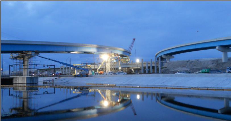
Construction of I-595; completed in 2014
