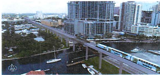
80-foot high-level fixed bridge
