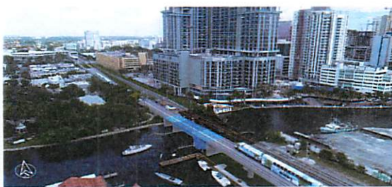
21-foot low-level bascule
