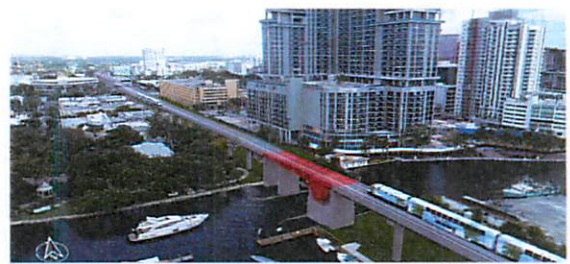
56-foot mid-level bascule
