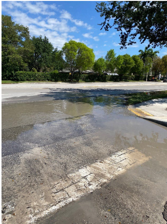
Flooding near construction site on eastern half of corridor.
