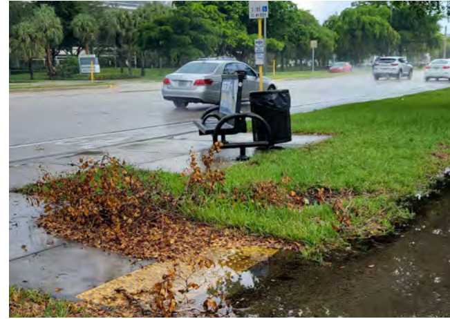
SB BCT Bus Stop north of Marcano Blvd: No shelter and no access to sidewalk on Access Rd
