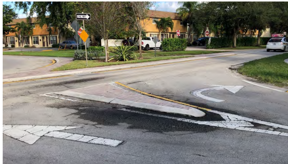
Intersection at NW 8th St, NW 46th Av, and NW 9th Dr (looking west), At this location, all west bound traffic is diverted north to NW 9th Ct.
