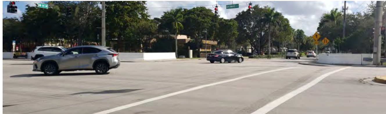
Broward Bl intersection (SE view); Inadequate pedestrian facilities and no left turn signals (on cross street).
