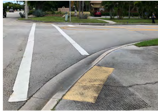
S. Marcano Blvd: The eastern ROW sidewalk ends. There is no signage for pedestrians to use sidewalk within NW 79 Te
