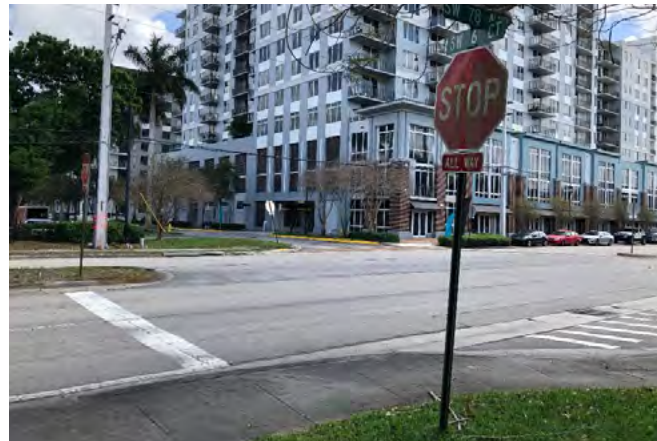
SW 78th Av and SW 6th Ct intersection (SE view). Minimal pedestrian features, including no crosswalk over northern leg.
