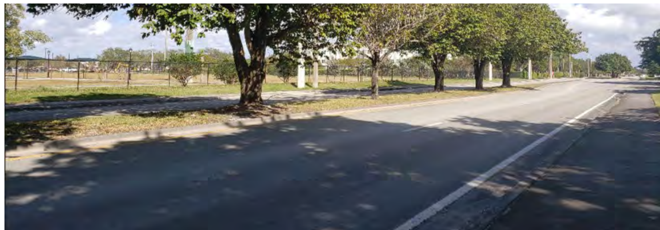
Western end of SW 6th St (east view). Sidewalks located at the curb. No pedestrian entrance to abutting Pine Island Park.
