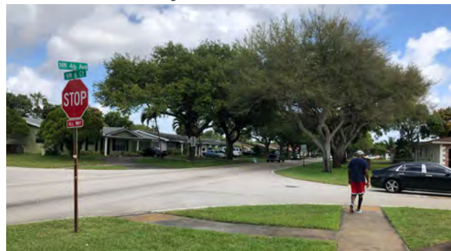
NW 6th Ct intersection (north view). Leads to Plantation Elementary School's pedestrian entrance but is missing high-visibility pedestrian features.
