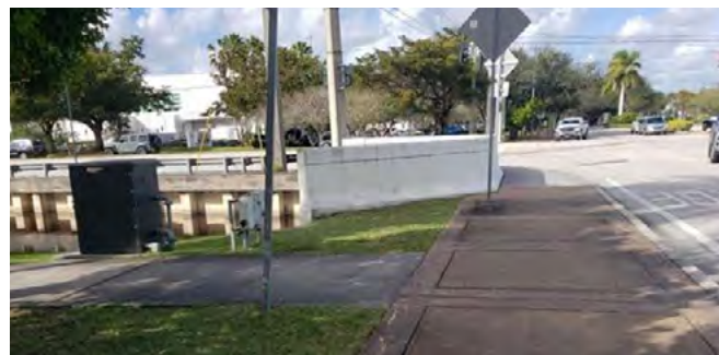
Greenway south of Broward Bl (western terminus at SW 84th Av). Connection over roadway is missing.
