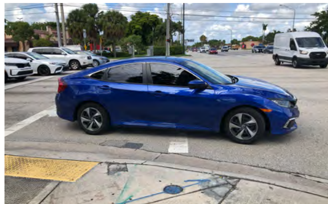
Sunrise Blvd: Above-ground utility in NW corner requires EB to SB right-turn vehicles to stop in crosswalk to see SB traffic.
