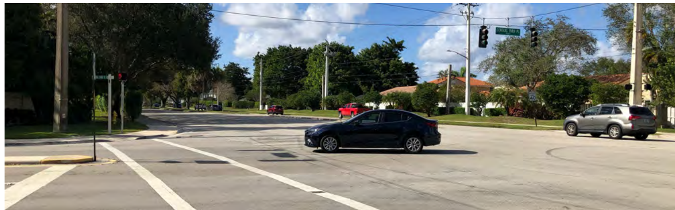
Central Park PI intersection (NW view). Minimal streetlights and no pedestrian-scale lights.
