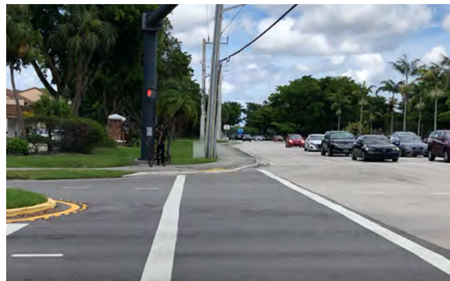
Cleary Blvd: One of the signalized intersections missing a crosswalk over University Dr.
