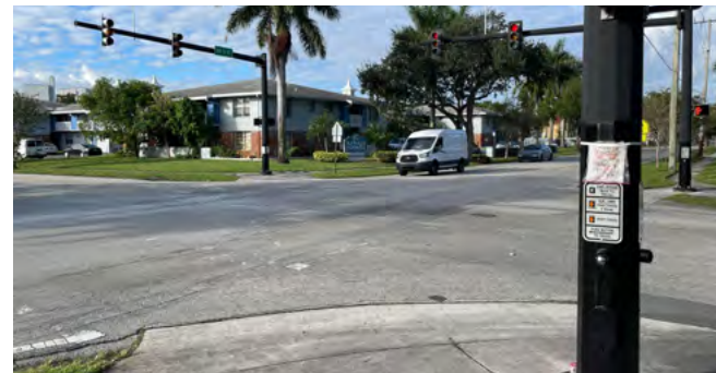
NW 42nd Av intersection (SW view); Low visibility crosswalks are worn out, detectable warning surfaces are missing, and there is no left turn signal.
