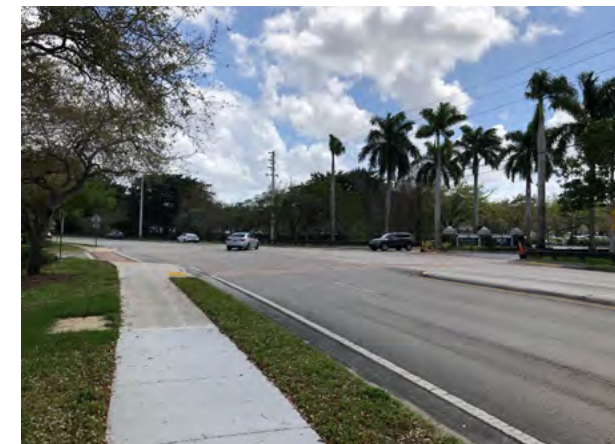
SW 78th Av – Entrance at Crossroads Office Park: Recommendation Group #1
