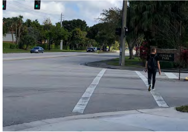
Central Park Dr intersection (East view). Low visibility crosswalks and no left-turn signals.
