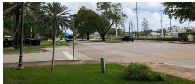
SW 3rd St intersection (SE view). Raised intersection with stop sign only on SW 84th Av. Pine Island Park abuts intersection.
