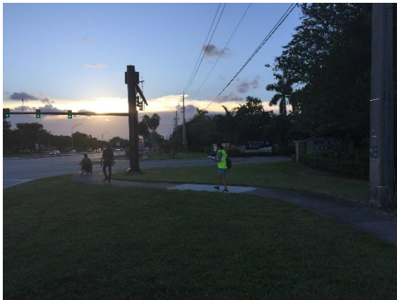
No pedestrian lighting along the study corridor.
