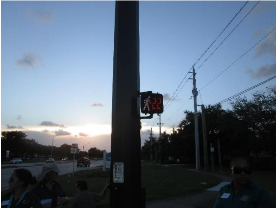
Evaluate the pedestrian signal timing to allow adequate pedestrian crossing especially at Oakland Park Boulevard and NW 68 th Avenue.
