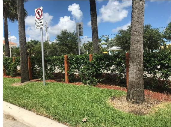
Consider installing a median treatment such as fencing with planter and vegetation at high pedestrian and bicycle volume locations to prohibit mid-block crossing.
