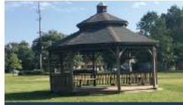
MISSING ACCESSIBLE ROUTE
