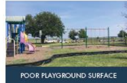
POOR PLAYGROUND SURFACE
