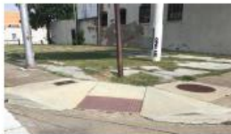
STEEP CURB RAMP RUNNING SLOPE
