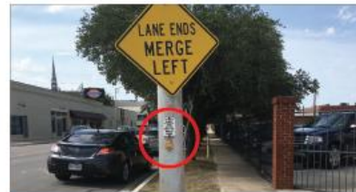
UNDERSIZED PUSH BUTTON (NOT TWO-INCH DIAMETER)
