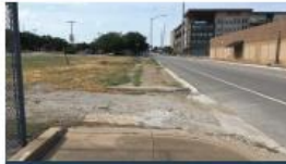
MISSING CURB RAMP
