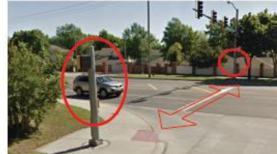
MISSING PEDESTRIAN SIGNAL AND PUSH BUTTON
