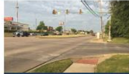
CURB RAMP GUTTER/TRANSITION
