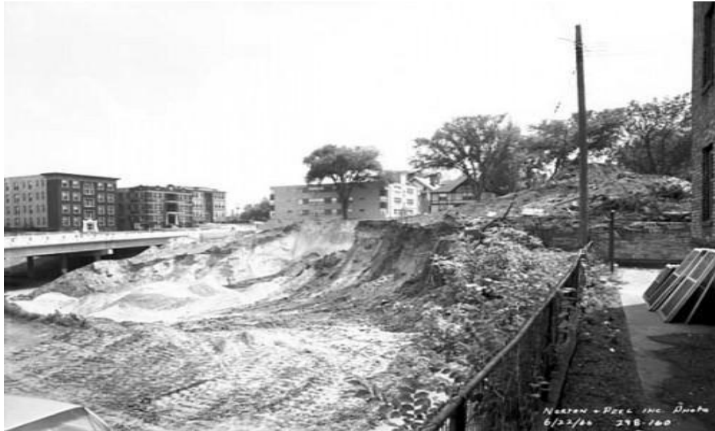
I-94 Construction through Rondo, 1966
